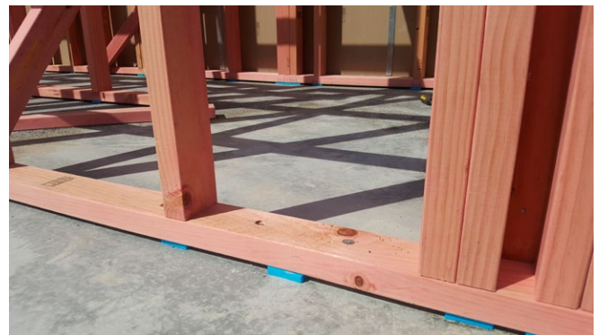
Bracing element showing additional bottom plate fixings and suggested additional packer on concrete floors.
